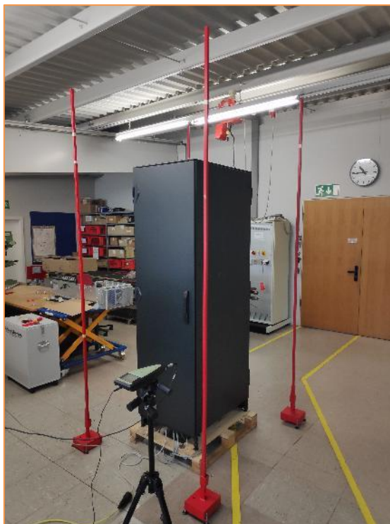
Figure 3 Noise measurement setup for LHX+ 5kW with closed doors_Rear view
