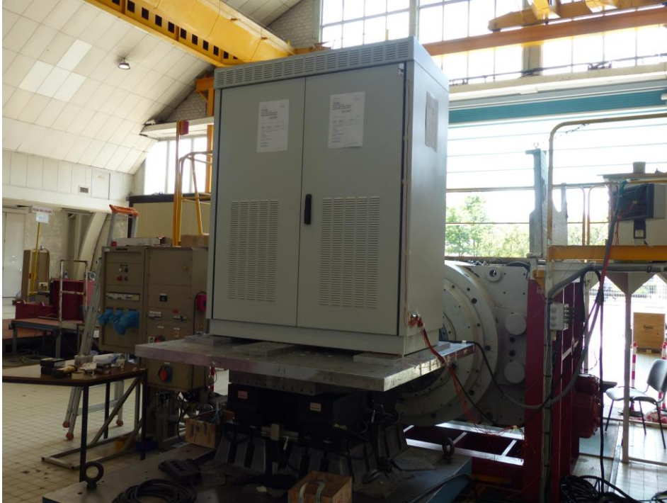
Photograph n°4 : Overall view along Transverse axis
