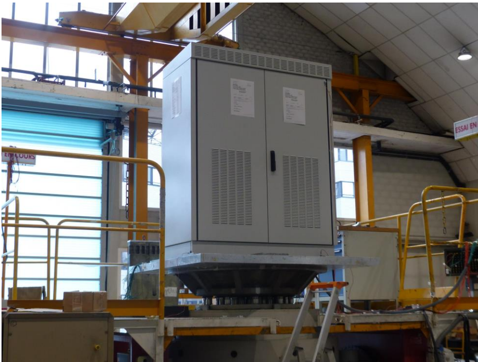
Photograph n°5 : Overall view along Vertical axis
